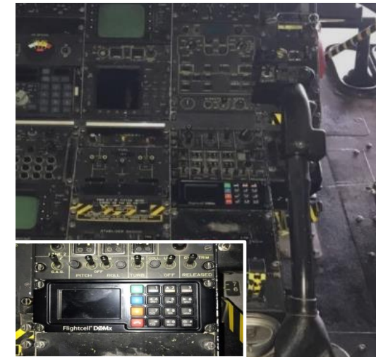
DZMx cockpit installation
